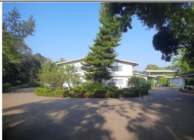
Factory front View
